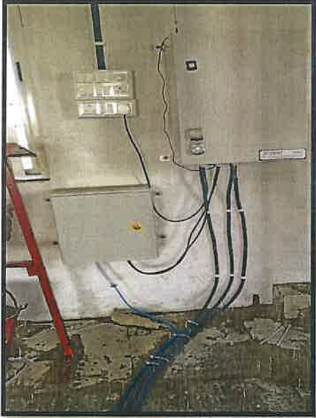
Location:- PUMPING STATION-C1
