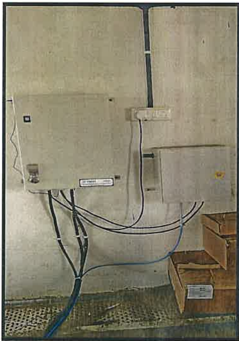
Location:- PUMPING STATION-C2
